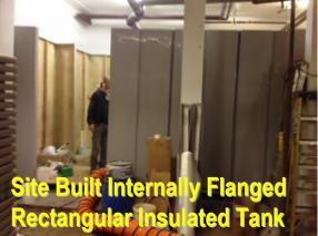
Site Built Internally Flanged Rectangular Insulated Tank
